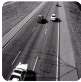
Figure 2. Loop detector
