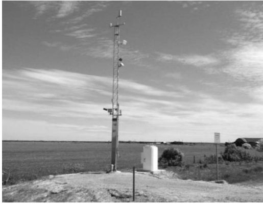
Figure 11. Environmental sensor stations
