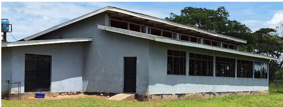
Fig. 2 The structure in Arapai—Busitema University where the experimental chickens were kept
